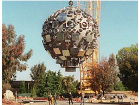
Figure 8.11. \sim 30 -foot diameter NIF main target chamber being position into facility. During operation, 192 high-power lasers focus on a target the size of a BB projectile to simulate and understand issues of nuclear fusion.
