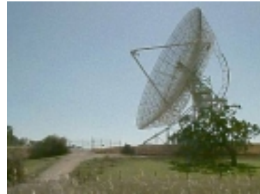
150 ft. diameter radio telescope dish for radar and communications Stanford University 1960s
